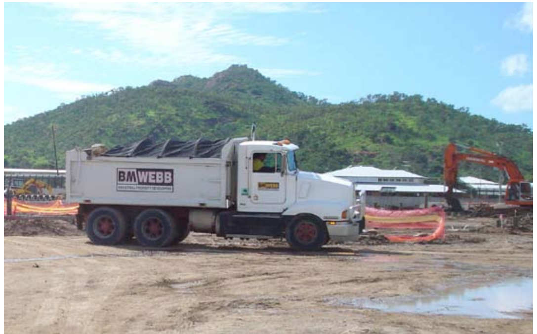
Construction work at the Cleveland Youth Detention Centre expansion
